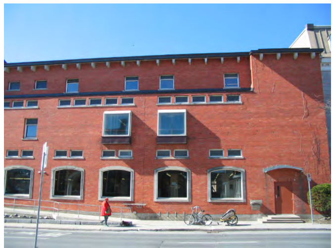
Northern portion of facade with small oriels and inset upper storey
