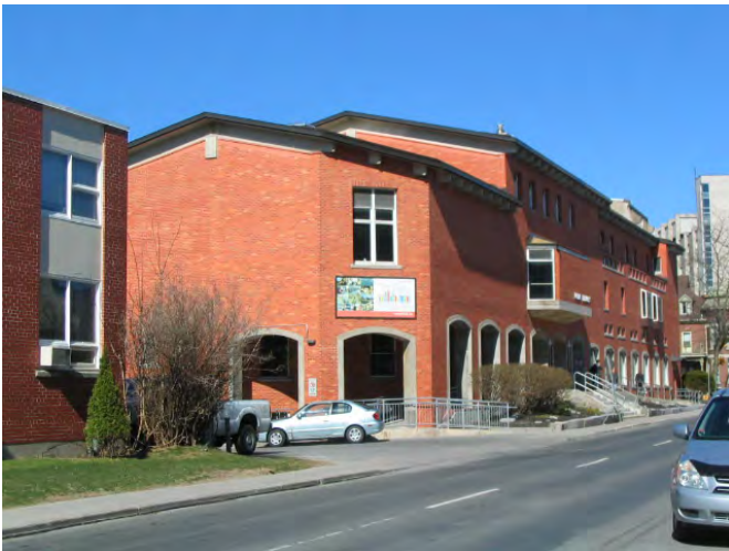
View of 1978 addition from Wellington Street looking north up Johnson Street
